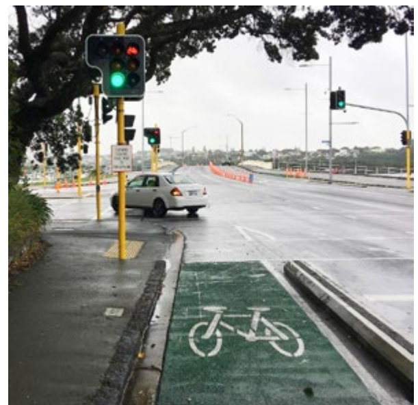
Figure 6-39c: Vehicles allowed to proceed left while MS lane users are held on red signal
