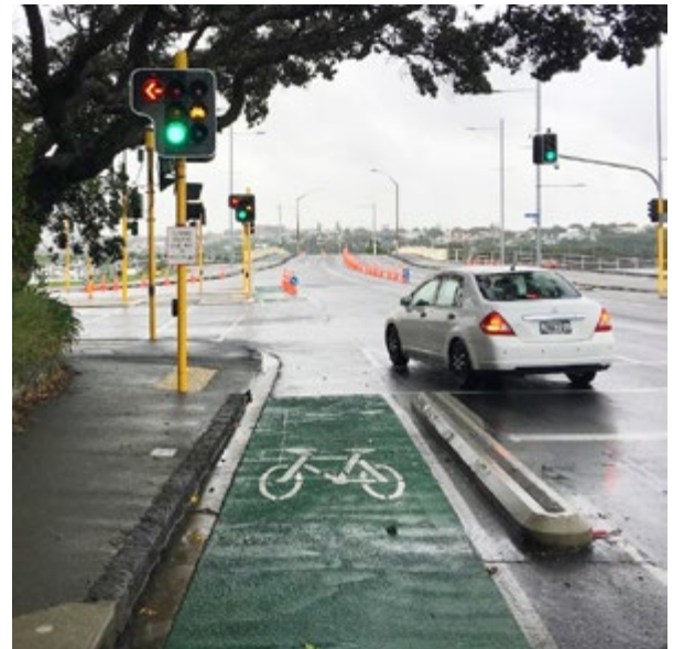
Figure 6-39b: Vehicles held from turning left and MS Lane users warned of signal change
