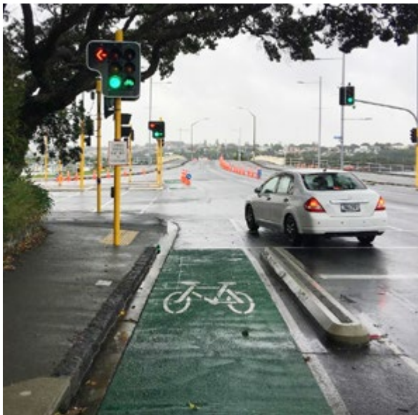
Figure 6-39a: Vehicles held from turning left so that MS Lane (cyclists here) can proceed
