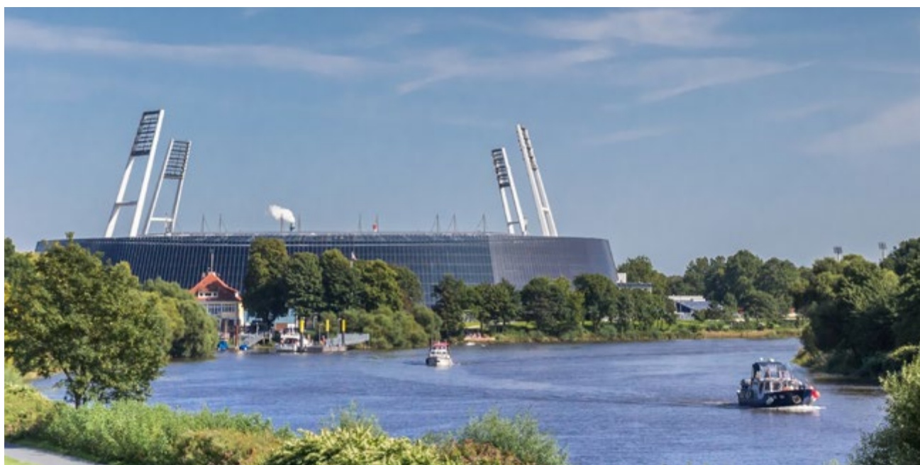
Figure 7 – Weser Stadium, Bremen, Germany – 6000m 2 or 200 000 photovoltaic cells cover the 40 000 seat stadium roof
