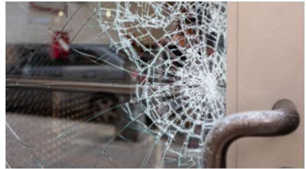
Figure 23 – Laminated glass to minimise secondary damage from glass shards caused by primary impact
