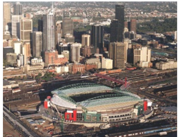
Figure 9 – Marvel Stadium Melbourne (then Colonial Stadium) – isolated and on its own
