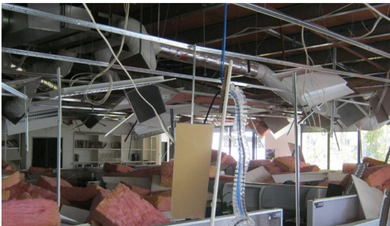
Fig 1: Aurecon Christchurch Office after the February 2011 earthquake showing extensive damage to suspended services and ceiling grid, (Image courtesy of Lee Howard, Aurecon Christchurch office)
