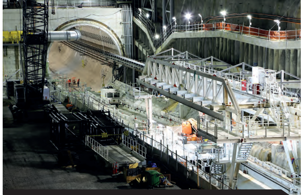
The 68m-long culvert gantry before installation in the tunnel
