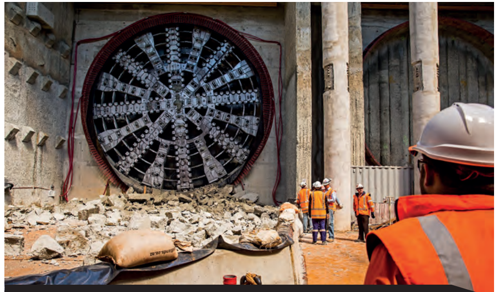
The tunnel's progress – breakthrough of the first tunnel at the end of September
