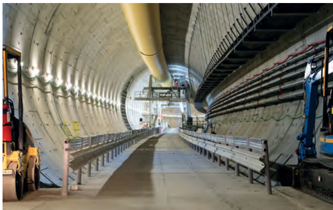
The culvert is being progressively backfilled with a road bed consisting of a 2.2m high culvert in the centre with sides filled with 40mm road base material to culvert level before a 1.2m high second stage backfill is placed on top
