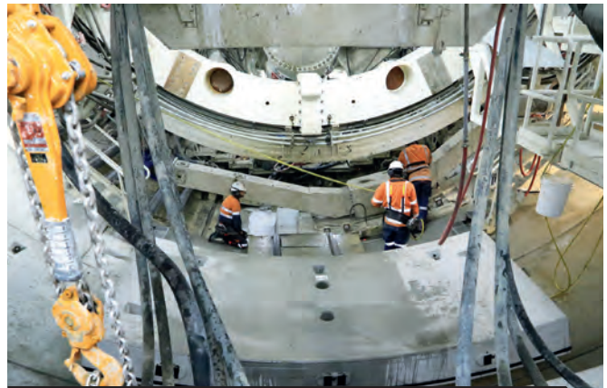
Segment erection on the TBM: the Waterview tunnels will be completely lined by 24,040 pre-fabricated tunnel lining concrete segments installed by an erector that picks up the segments that enter the TBM via a gantry and installs them one at a time
