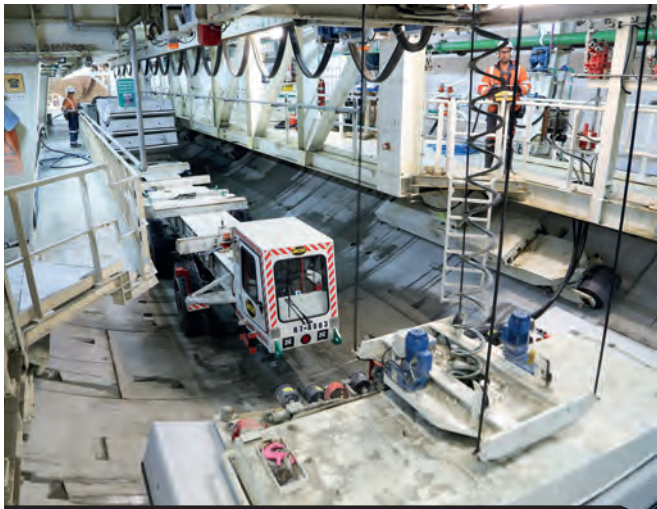
Segment delivery to the TBM by means of a special trailer
