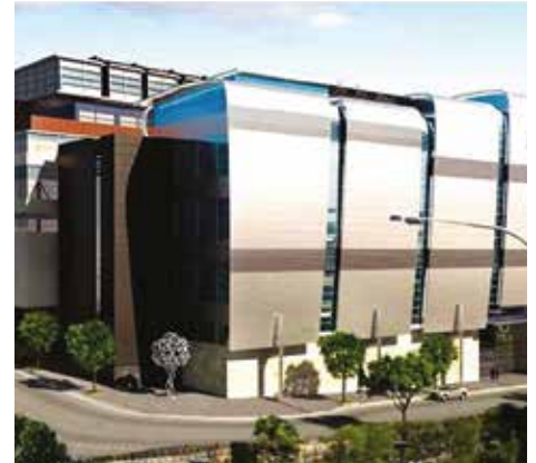
Global Switch East and West Data Centres Australia
